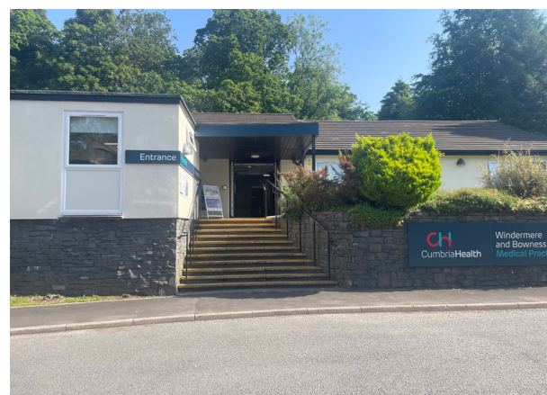
External view of building
